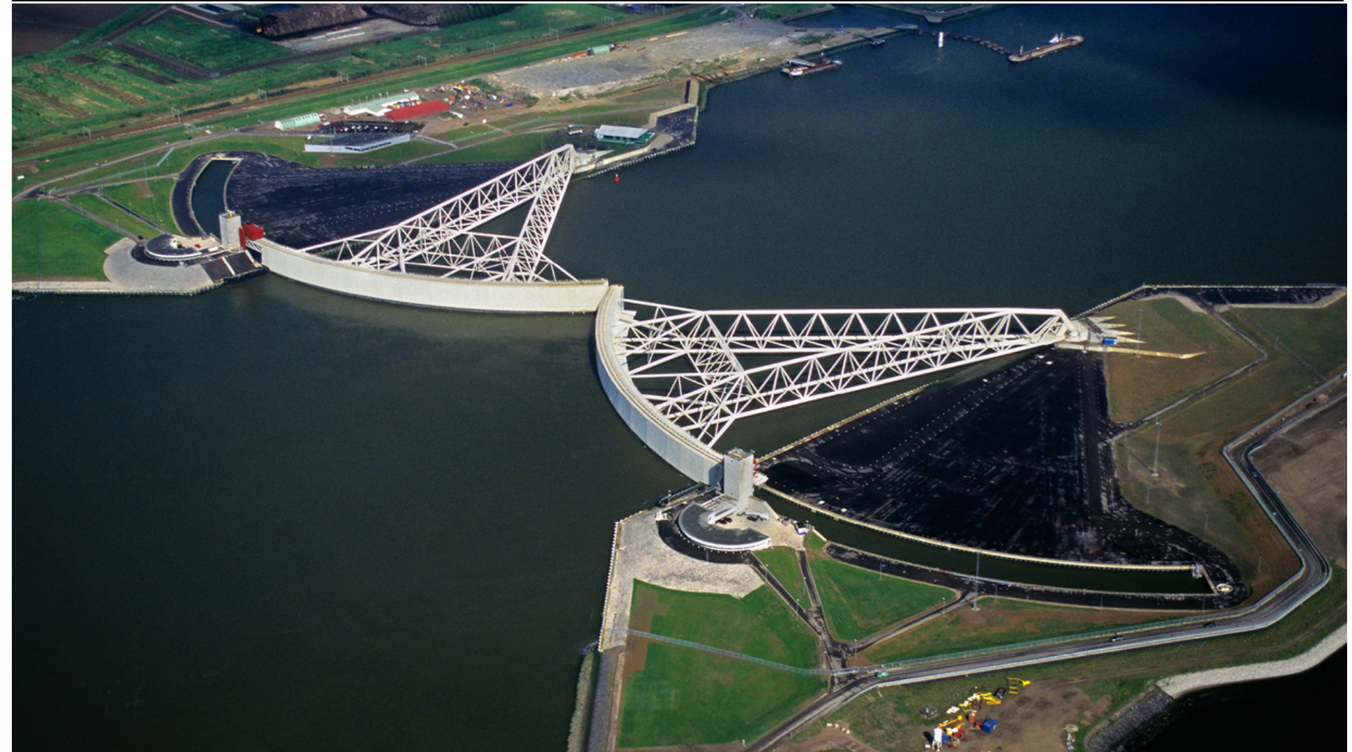
The arms of the Maeslantkering storm barrier
